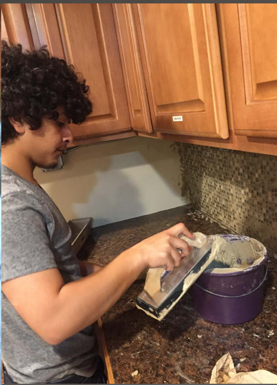
Grout Installation
