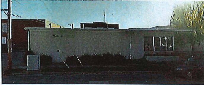
(Front Exterior - Street View)
